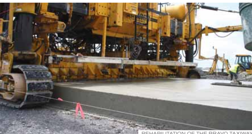
REHABILITATION OF THE BRAVO TAXIWAY
