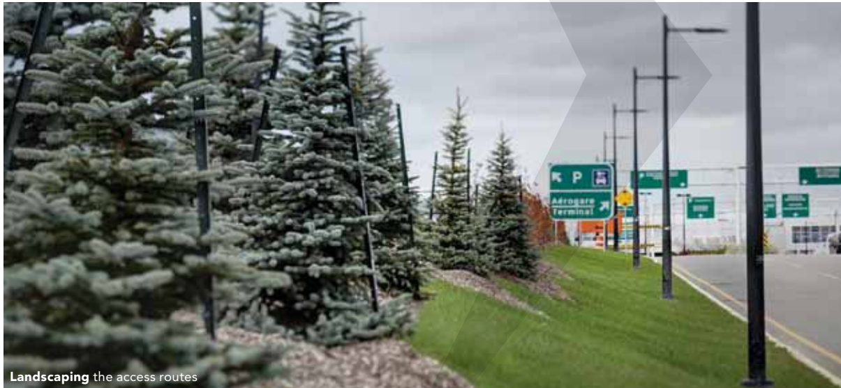
Landscaping the access routes
