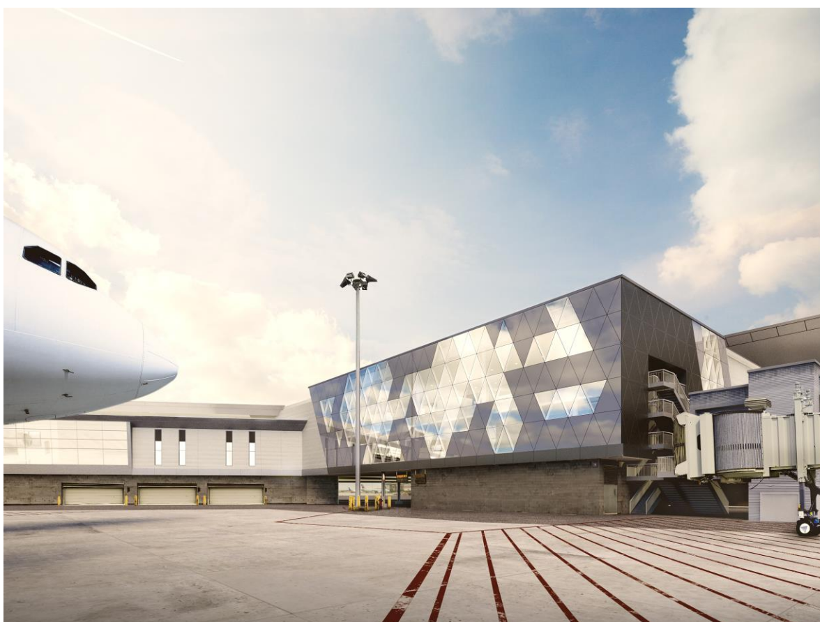
Connection Centre outside view
