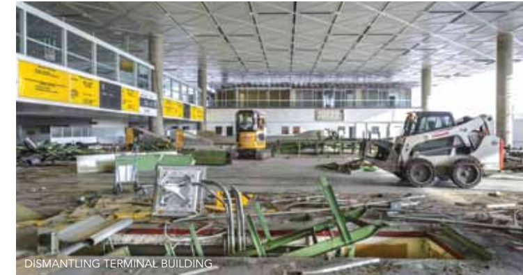
DISMANTLING TERMINAL BUILDING
