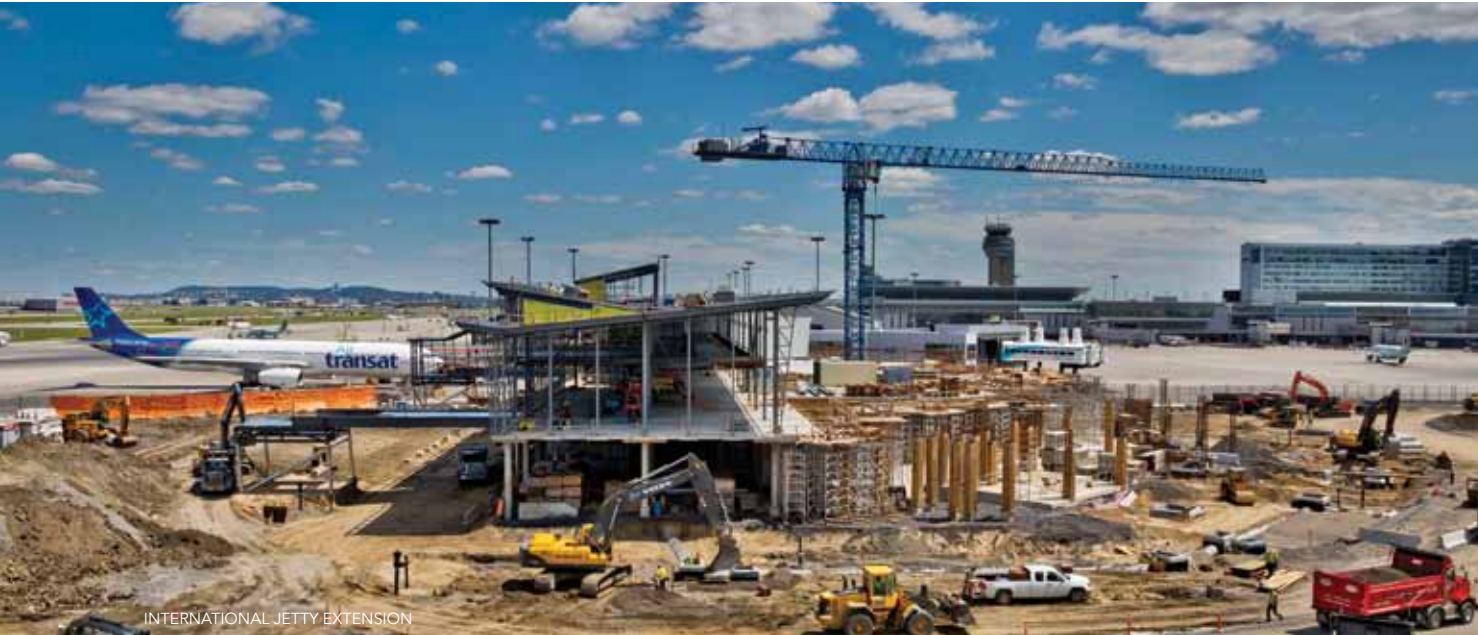
INTERNATIONAL JETTY EXTENSION
