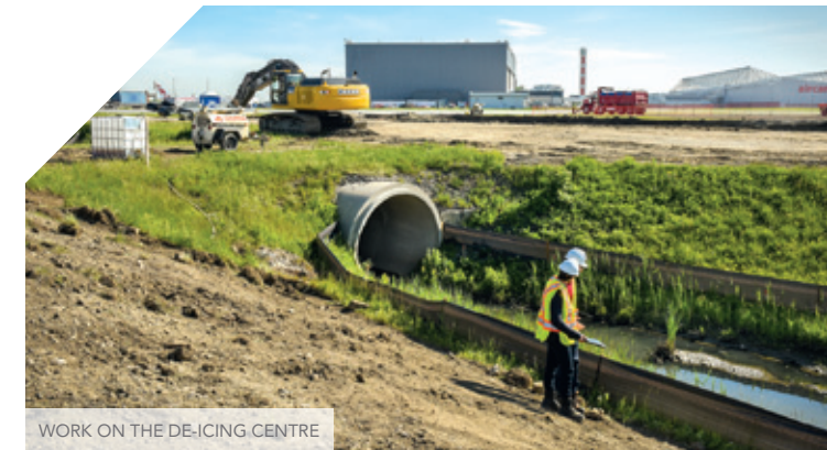
WORK ON THE DE-ICING CENTRE
